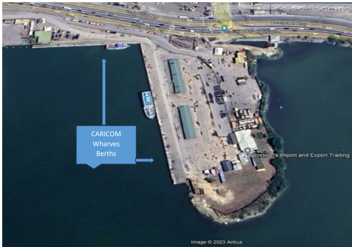
Figure 31. Port of Port of Spain – Queens Wharf - CARICOM Wharves area
